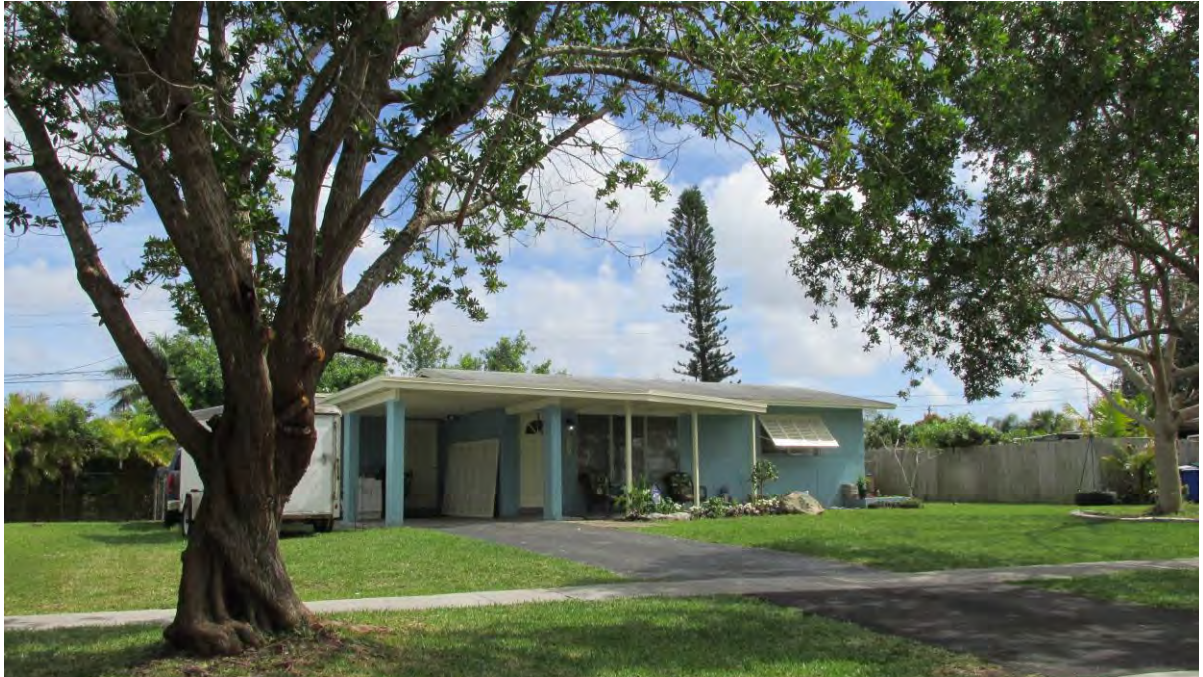
Figure 1. – Front (west elevation) view of 1624 East Lake Drive, Margate, as viewed today.
