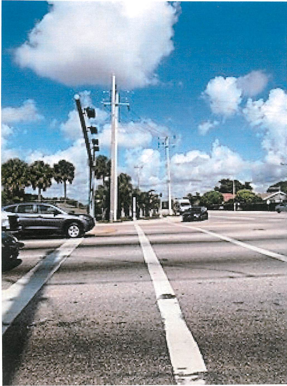
SW corner of Rock Island Road and Commercial Boulevard.
