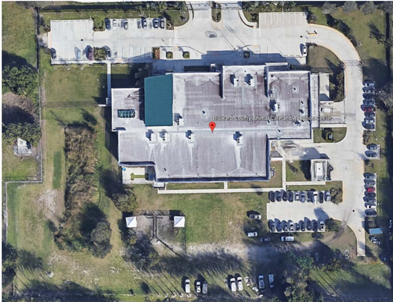
Figure 25 - Aerial View of ACAD Showing Parking from Google Earth
