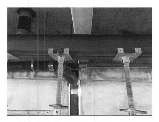
Exhibit 4: Cracked Haunch and Shored Joist below third floor.
