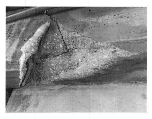
Exhibit 3: Cracked Haunch below third floor joist – No longitudinal rebar found here.
