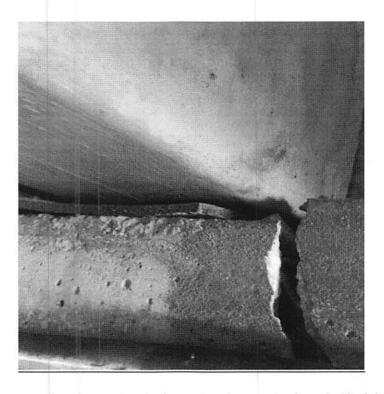
Exhibit 11: Loose bearing pad. Joist is not bearing on the front half of the cracked haunch.
