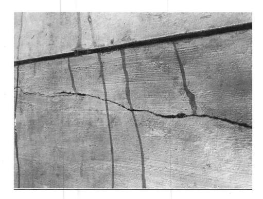
Exhibit 18: Slab cracks along the sides of a soffit beam.
