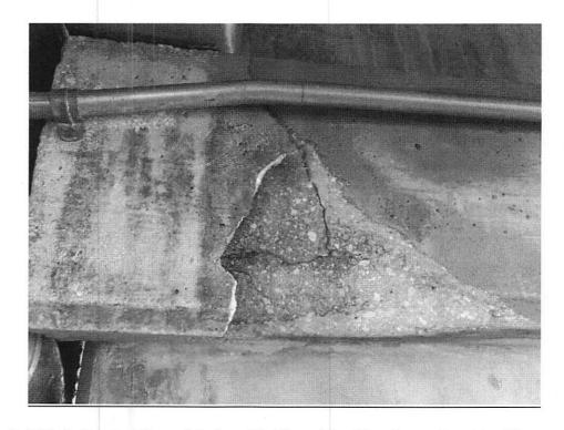
Exhibit 2: Cracked Haunch below third floor joist. No stirrups found in this area.
