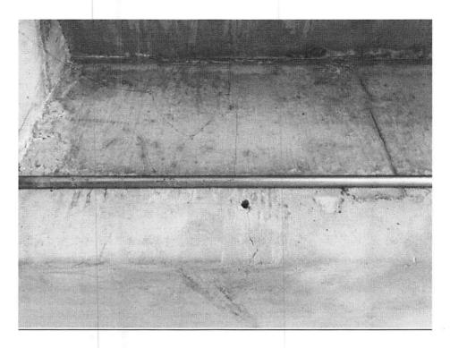
Exhibit 17: Vertical and diagonal cracks on a soffit beam.
