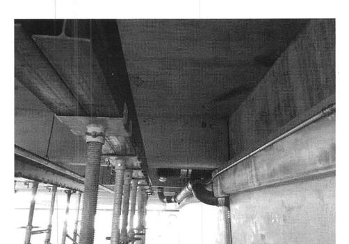
Exhibit 7: Steel beam and shoring detail at the top of shoring towers.
