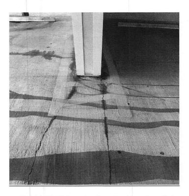
Exhibit 20: Slab cracks along the sides of a soffit beam.
