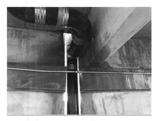
Exhibit 9: Condition where a third floor joist is at the edge of a haunch. Shoring is required here.
