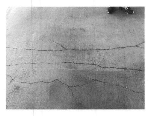
Exhibit 19: Slab cracks along the sides of a soffit beam.
