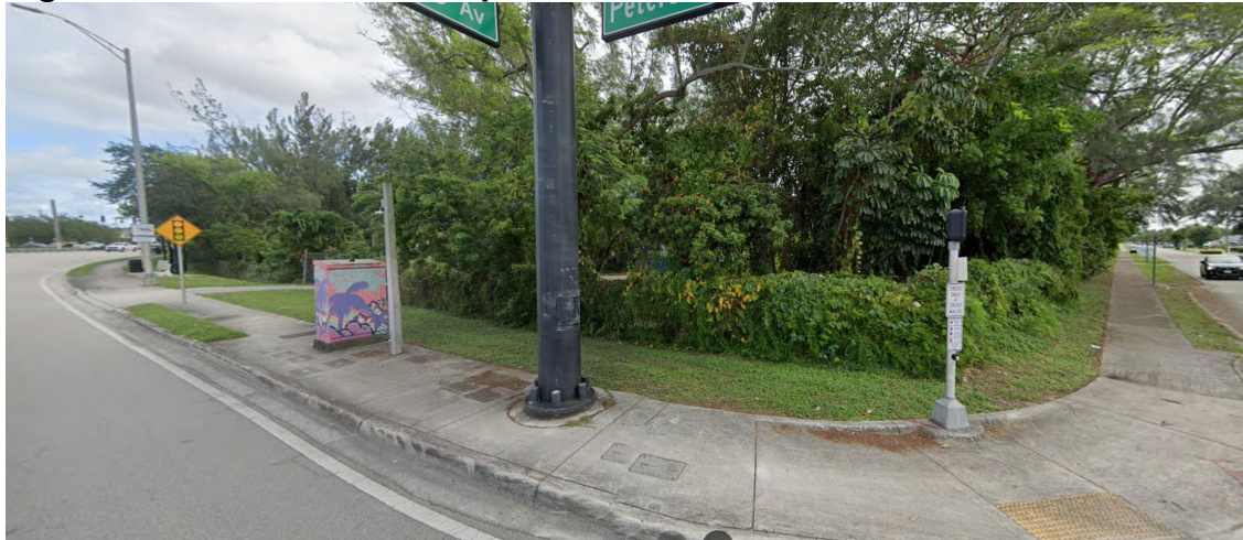
Figure 10: Sidewalk-Bus Stop Access Obstruction
