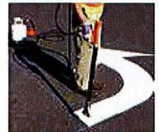
Fig. 3 Heat PreMark® material according to instructions.
