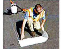
Fig. 2 Position PreMark® material according to diagram provided
