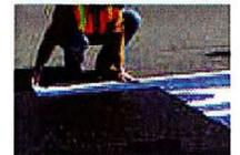
Fig. 6 Position PreMark® material according to diagram provided.
