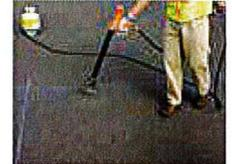
Fig. 1 Prepare area by removing debris with blower then remove moisture with heat torch
