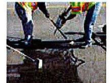
Fig. 5 Squeeze out sealer and spread with roller.
