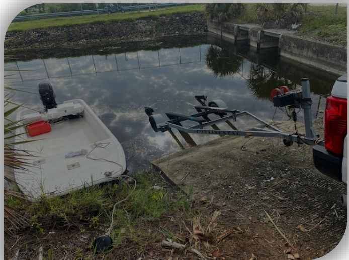
Equipment and Boat Ramp, Embankment, and Culvert Infrastructure
