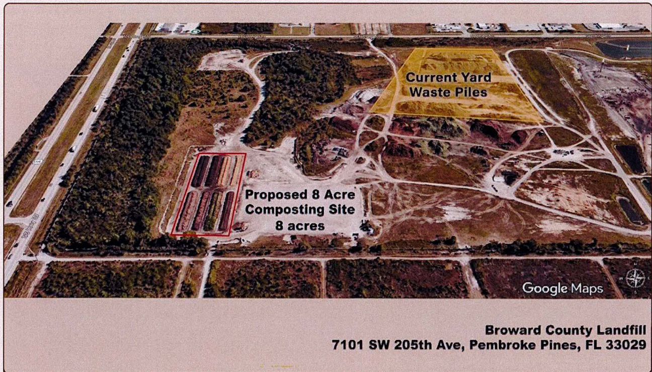
FIG. 02 — SITE ORIENTATION · BROWARD COUNTY LANDFILL · 7101 SW 205TH AVE, PEMBROKE PINES, FL 33029
