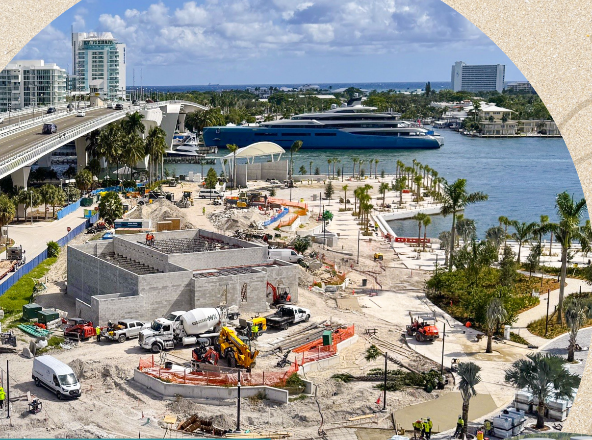
WATERFRONT PLAZA & AMPHITHEATRE (UNDER CONSTRUCTION)
