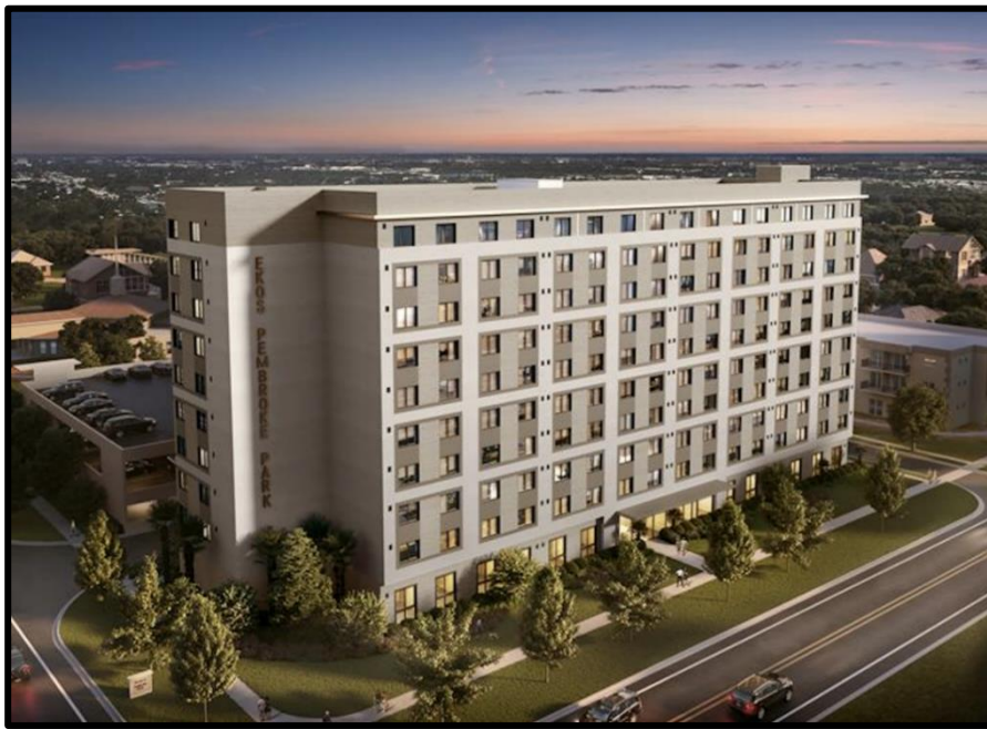
EKOS PEMBROKE PARK | 5595 SW 41 st Street, Pembroke Park A Live Local Act project with 150 multifamily units restricted to seniors making up to 605 AMI. The project was issued multifamily bonds totaling about $34.1M from the Broward County HFA.
