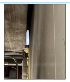
Image 11: Opening In Exterior Wall with visible daylight at PBB Penetration as viewed from ceiling above Unoccupied Space
